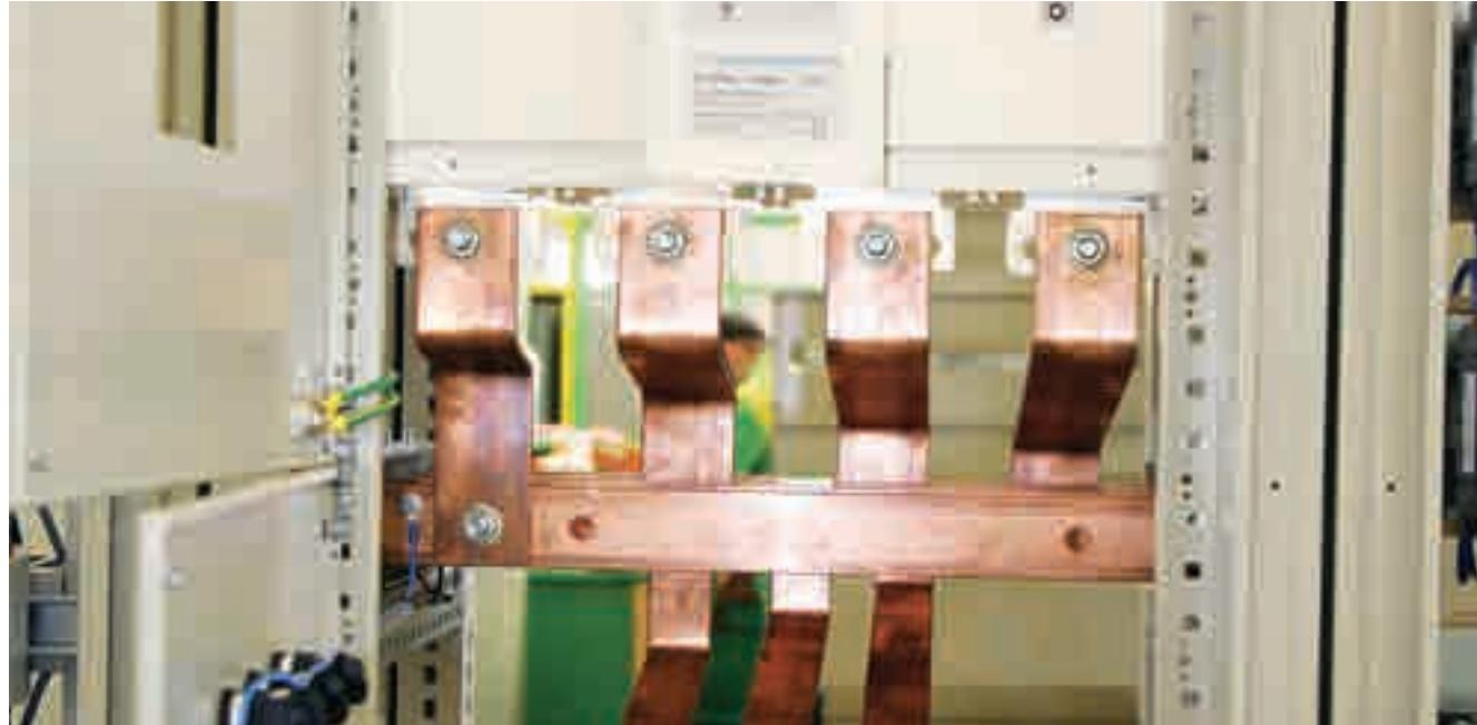
General low voltage panels, open, typically installed inside the compact substations. Can manufacture a diverse range of solutions, with circuit breaker or the switch input, outputs triple blocs, circuit breakers or fuser blocs.
